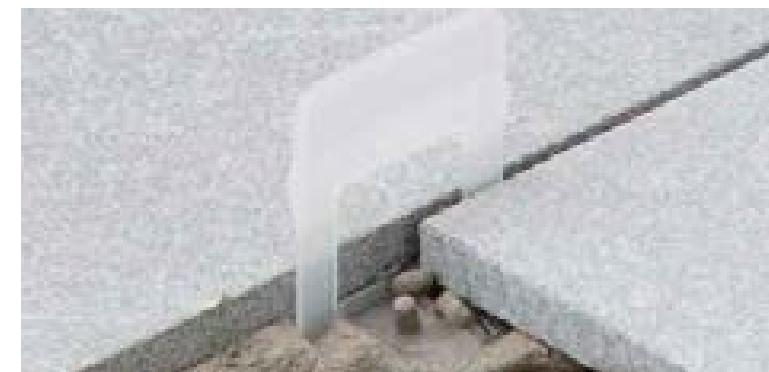
1. After spreading the adhesive cement, insert the clips underneath the tiles on all four sides.
